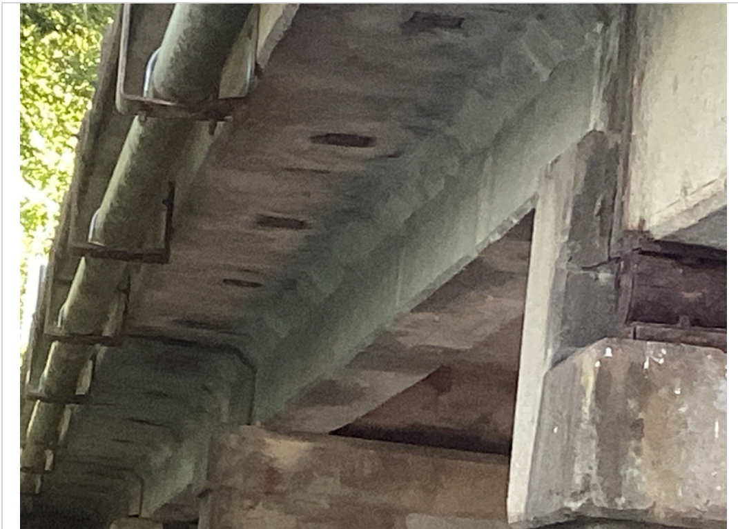
Crack repairs to beam "A" span #7
