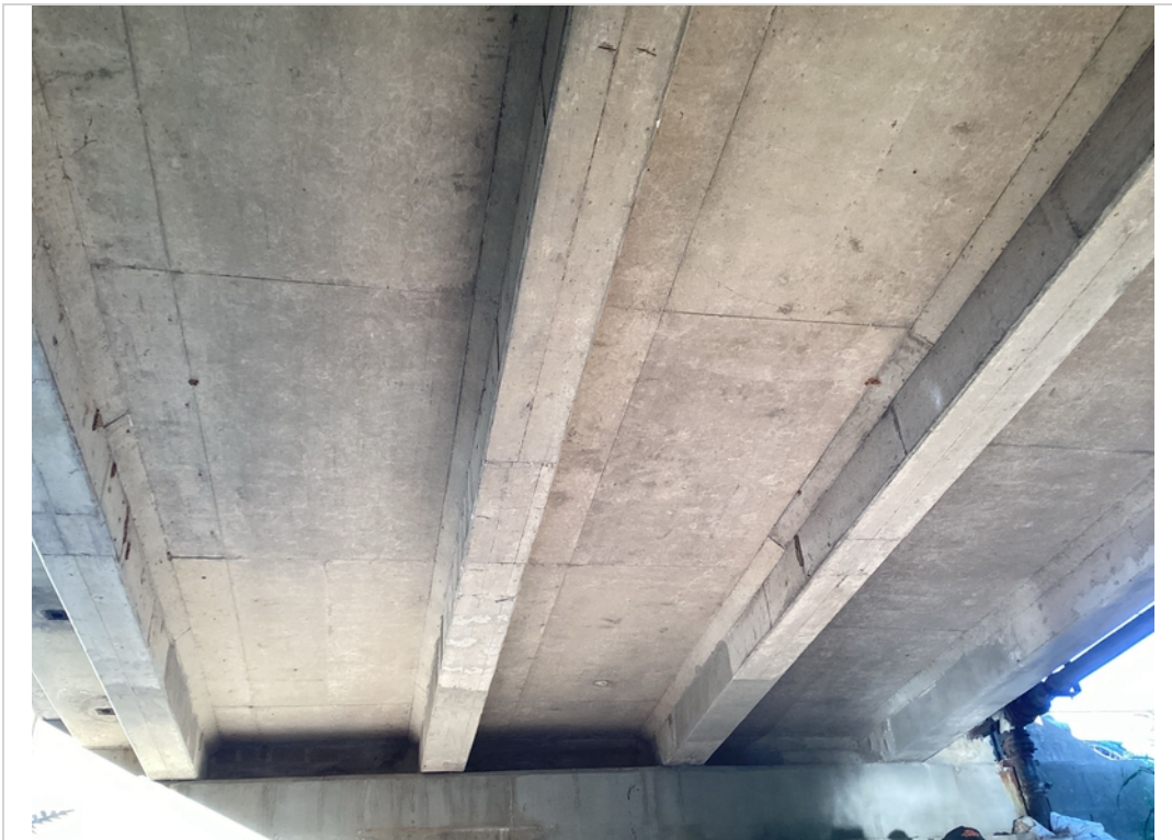
Repaired bottom of superstructure span #1, typical all
