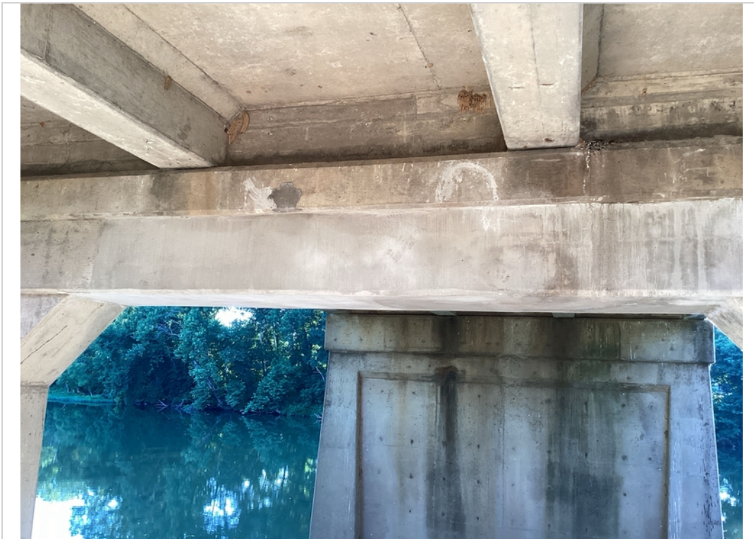
Bent caps have been repaired with new concrete
