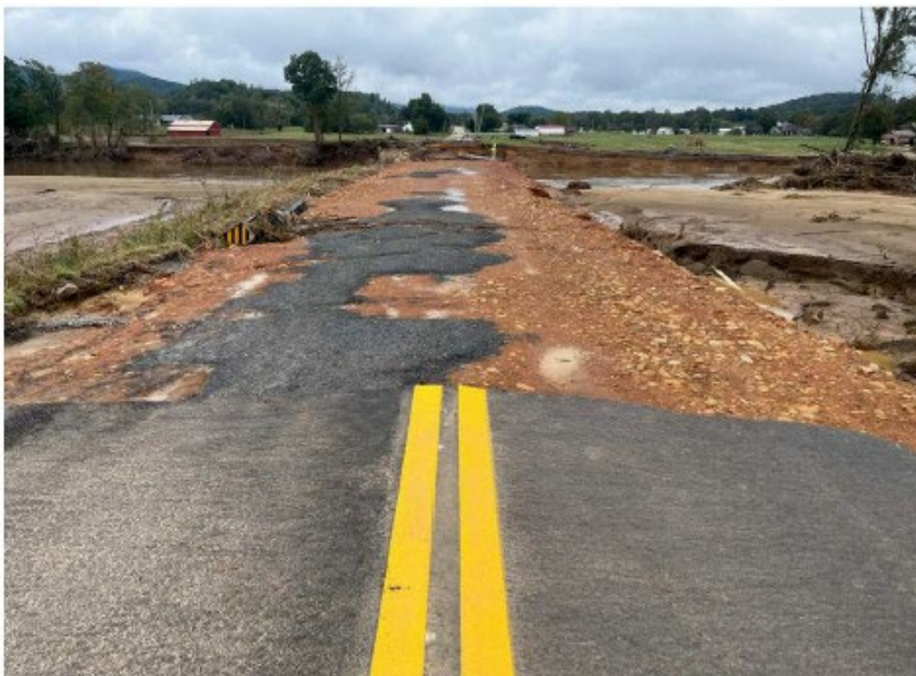
Figure 6: Damaged roadbed on the north side of the river looking south towards bridge location.
