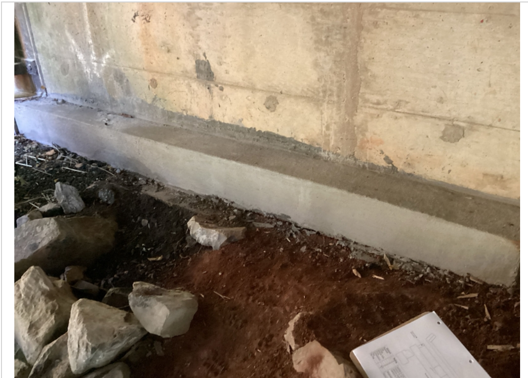
Previous settlement at abutment #2 has been repaired with a concrete cap
