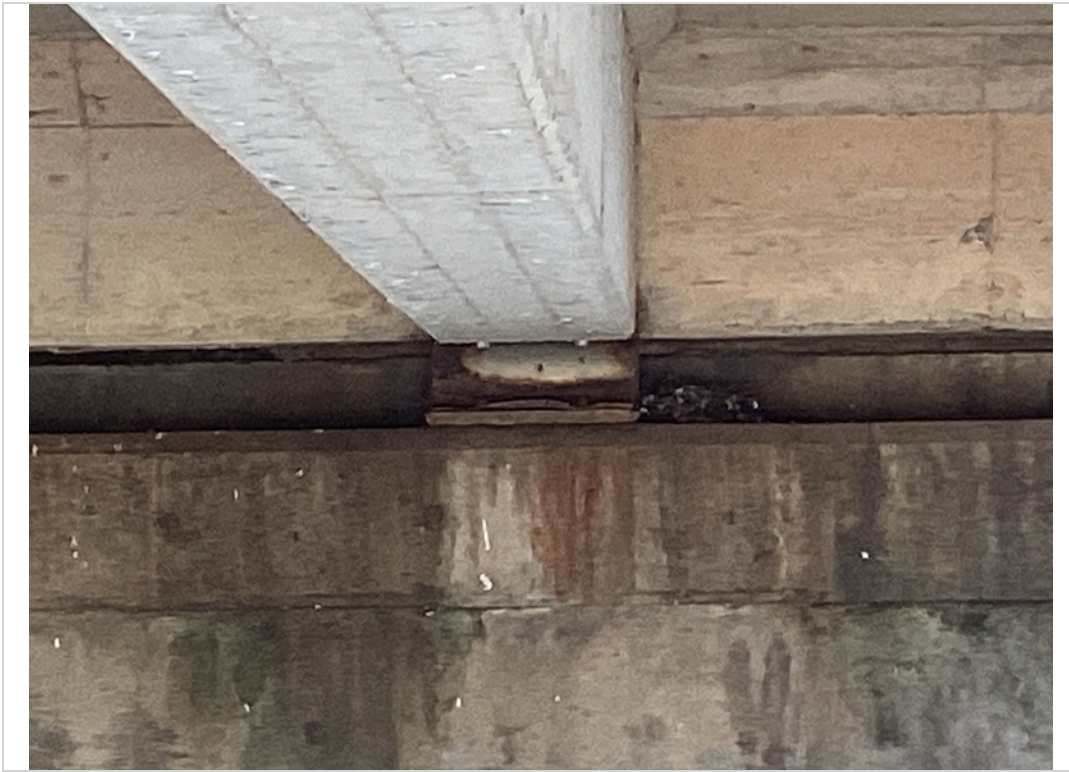
Heavy corrosion, flaking, pitting & section loss bearings spans #3 - #6
