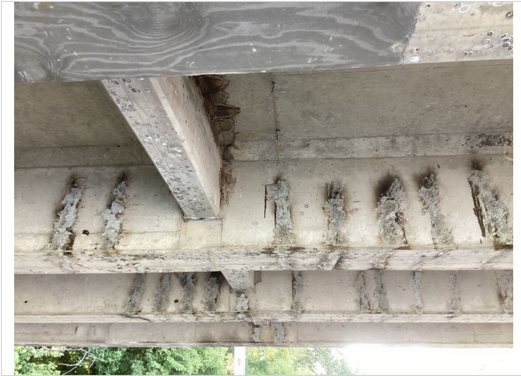
Crack repairs to beams "B, C, & D" span #6
