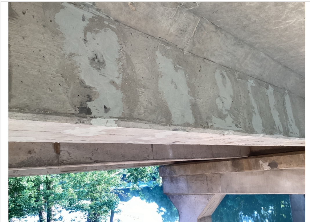
Repairs to vertical and transverse hairline to 1/8" cracks in all spans
