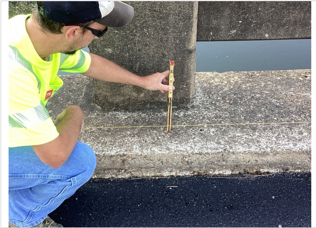
1.5" dead load deflection span #6
