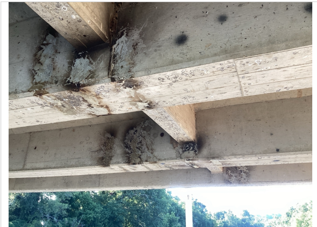
Crack repairs to beams in span #4
