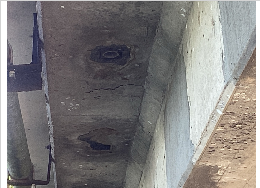
In place spall/delamination in left overhang span #1
