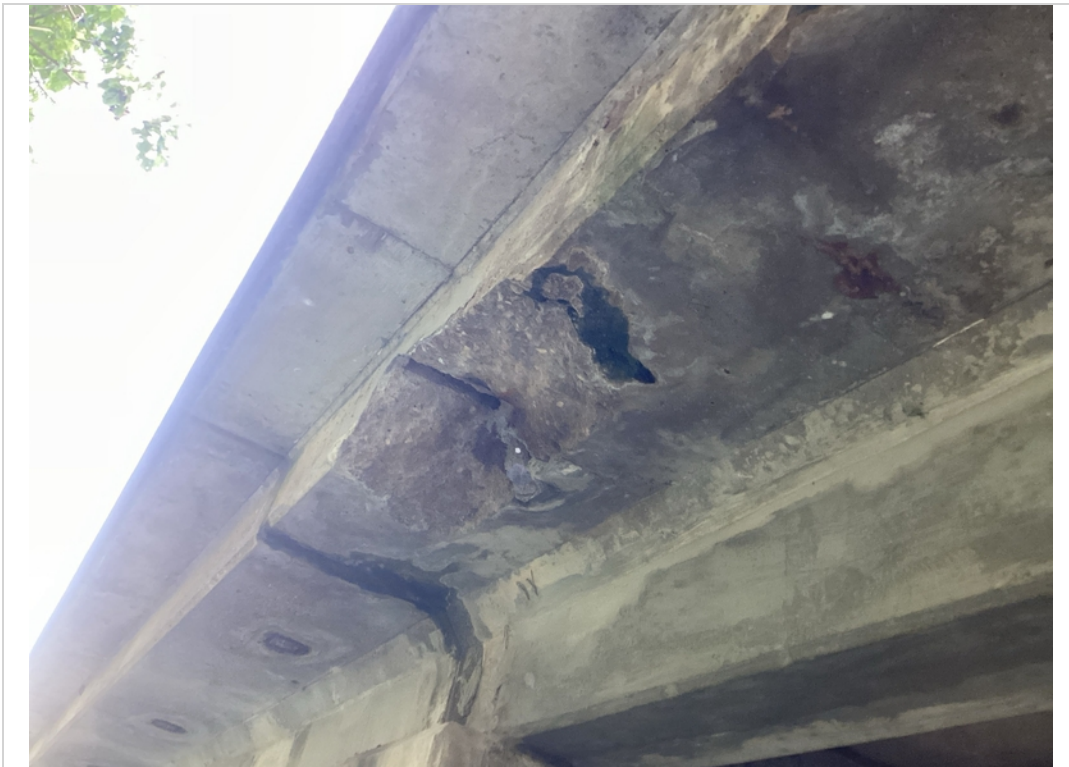
Span #9: Heavy spalling right side overhang
