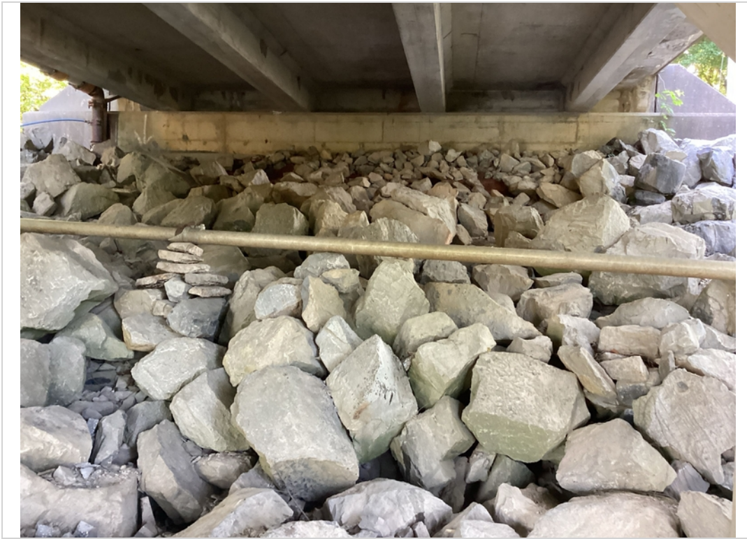
Shot rock added to abutment #2 bank
