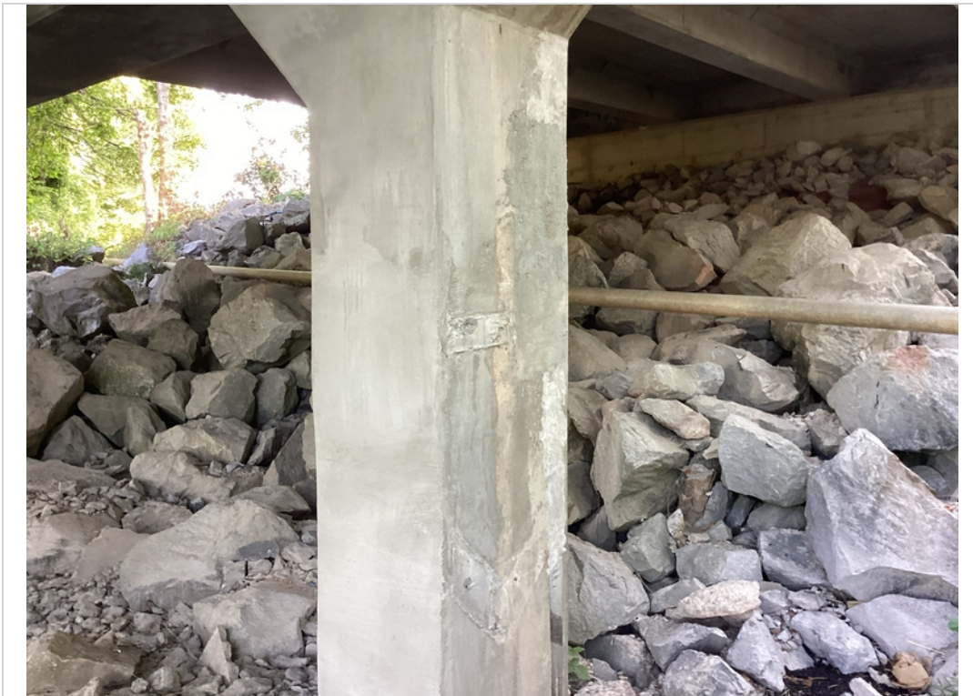
Cracking and spalls in bent columns have been repaired
