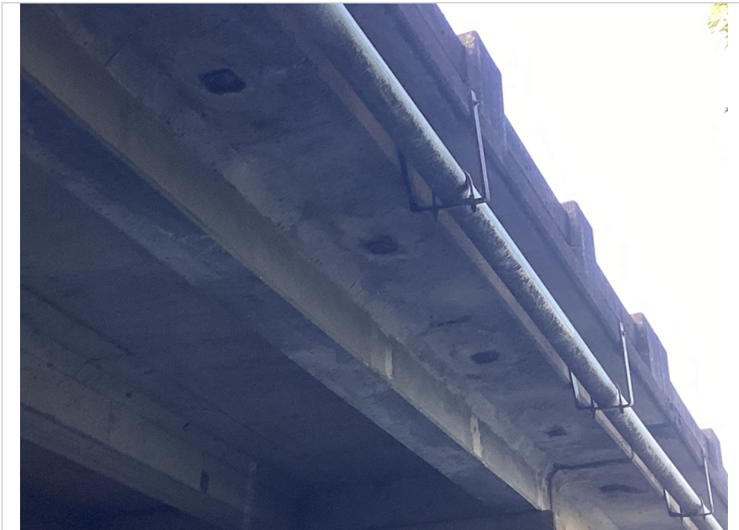
Repairs to spalling around drains all spans
