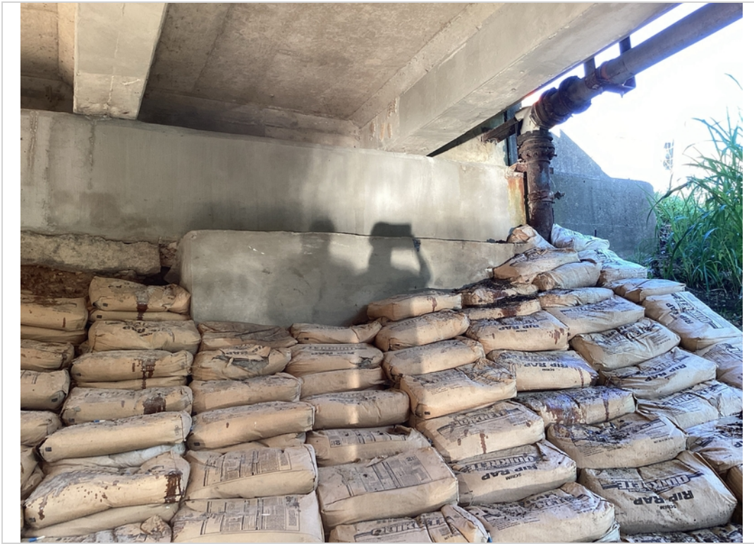
Previous void at abutment #1 has been repaired with a concrete cap, rip rap added to bank
